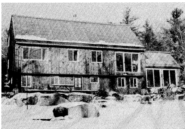
This solar home uses two 4000-gallon water tanks for heat storage.
